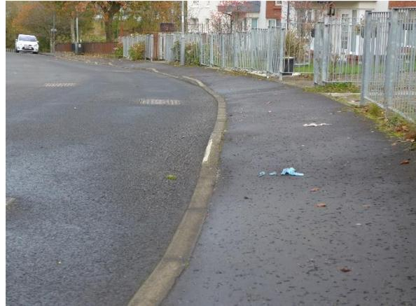
Excessive crossfall across whole footway. Lengthy sections of footway lacking a kerb detectable with a long cane.
