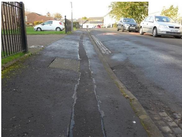
Excessive crossfall to support vehicle access
