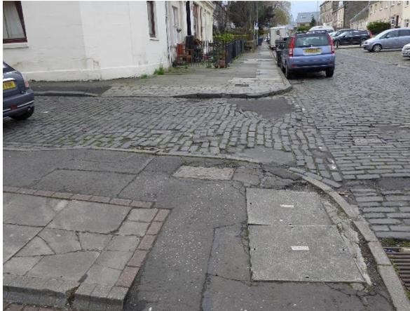
Poor surface. Break in footway continuity for minor access. Poor surface on minor access.
