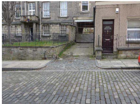
Break in footway continuity for minor access which appears unused. Poor surface on minor access.
