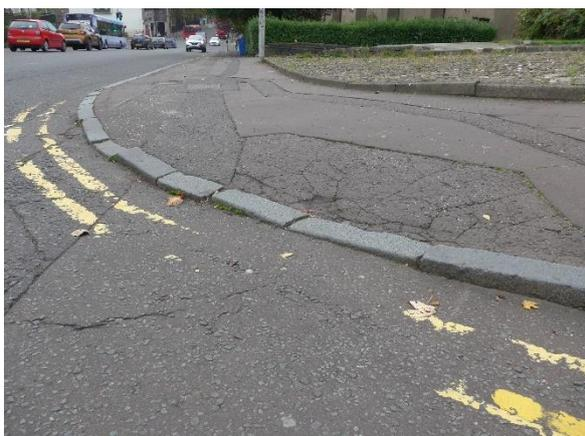
Close up detail from above-right photo, showing low kerb without tactile paving warning.
