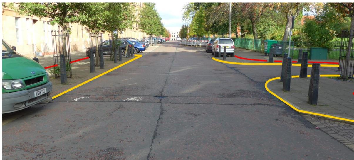
Photo 4: Footways built out both into side road and larger road (Govanhill). Red lines indicate position of original kerbs. Yellow lines highlight position of current kerbs.
